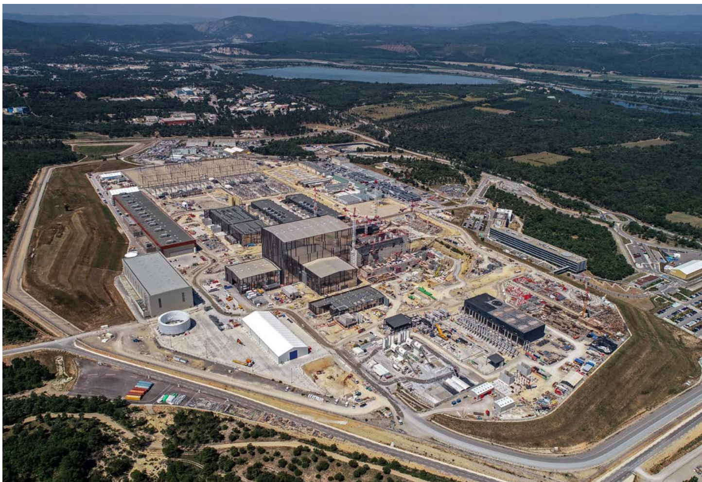
ITER: civil engineering work on the Tokamak Building, Cadarache (France)
