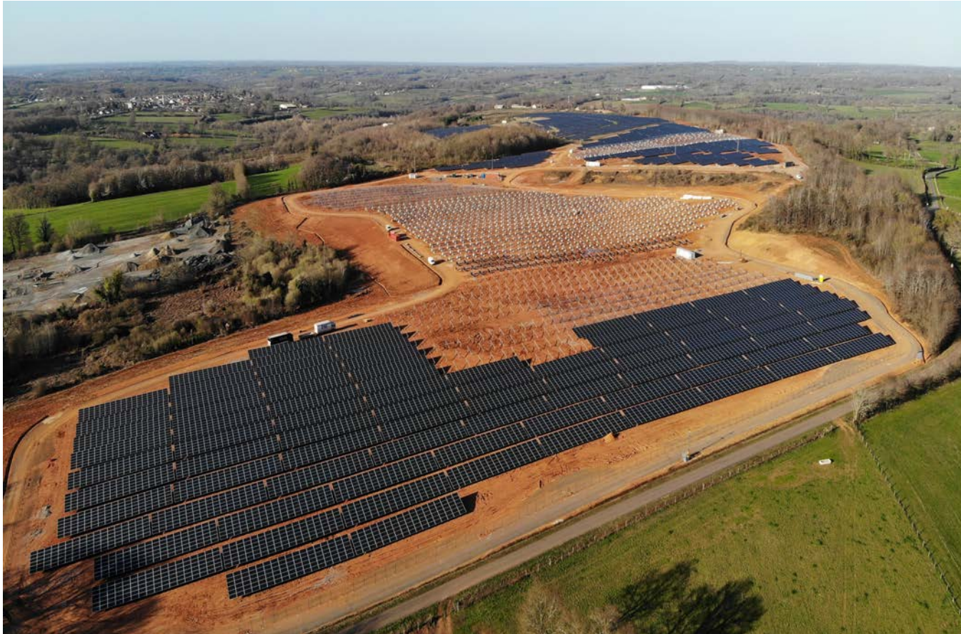
Solar power plant in Chaillac (France)
