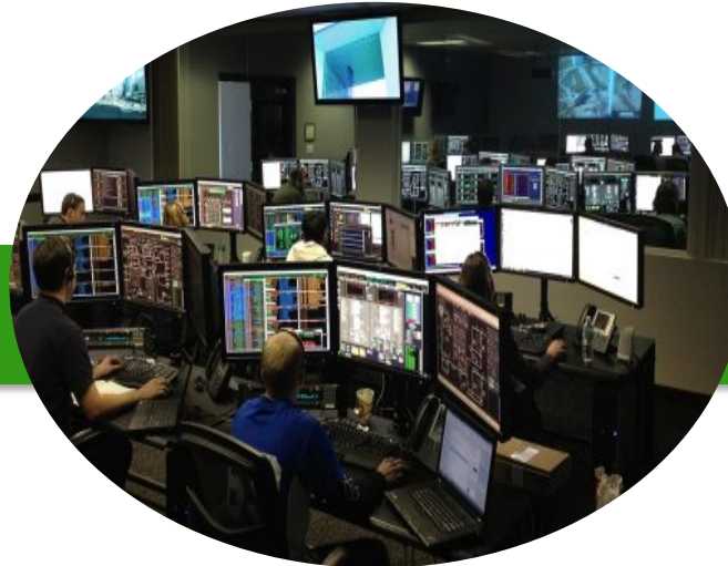
VINCI Energies: hypervisor platform at La Défense
