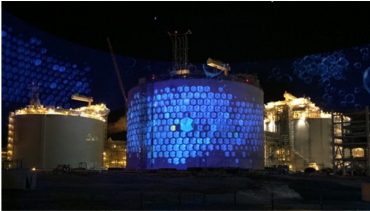
VINCI Construction delivers in December 2017 the Yamal LNG tanks, in Siberia
