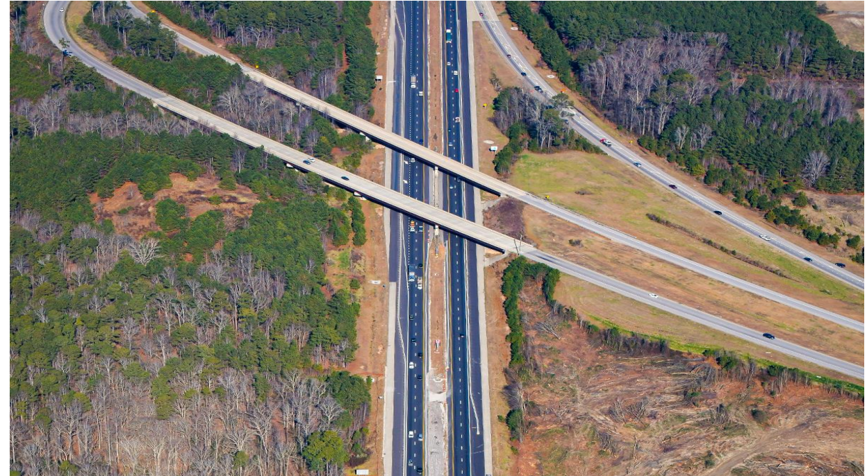
N.C. 540 Triangle Expressway in North Carolina (US)
