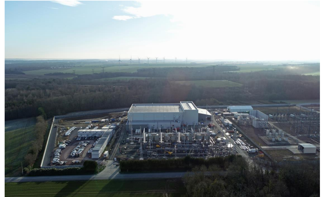
AC/DC converter station (Normandy) of the 230-km interconnector between southern England and northern France
