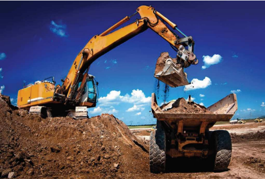
Optimize management of excavated materials
