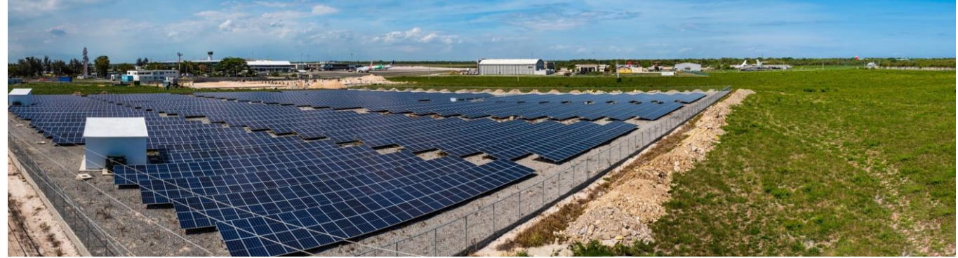
Installation of solar energy production capacity – VINCI Airports
